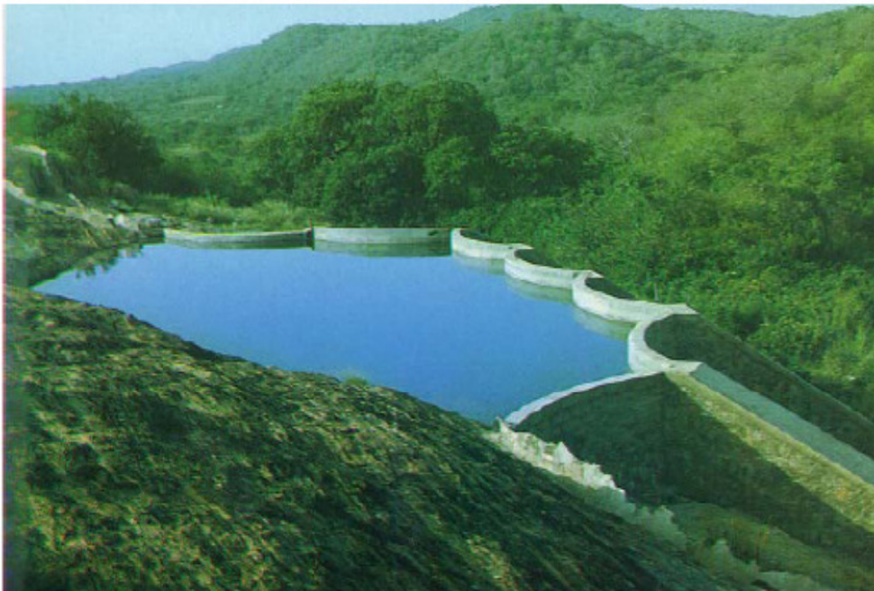
Figure 5: A masonry dam impounding surface water in Kenya
