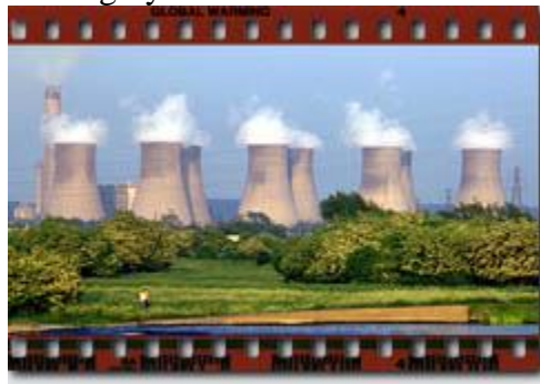
Nuclear power plants have had success in Europe, but not in the United States www.envirolink.org/orgs/edf/sitemap.html
