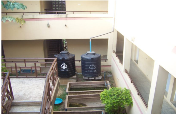
Figure 21: Rain harvester and repaired fibre glass tanks at AQFM
