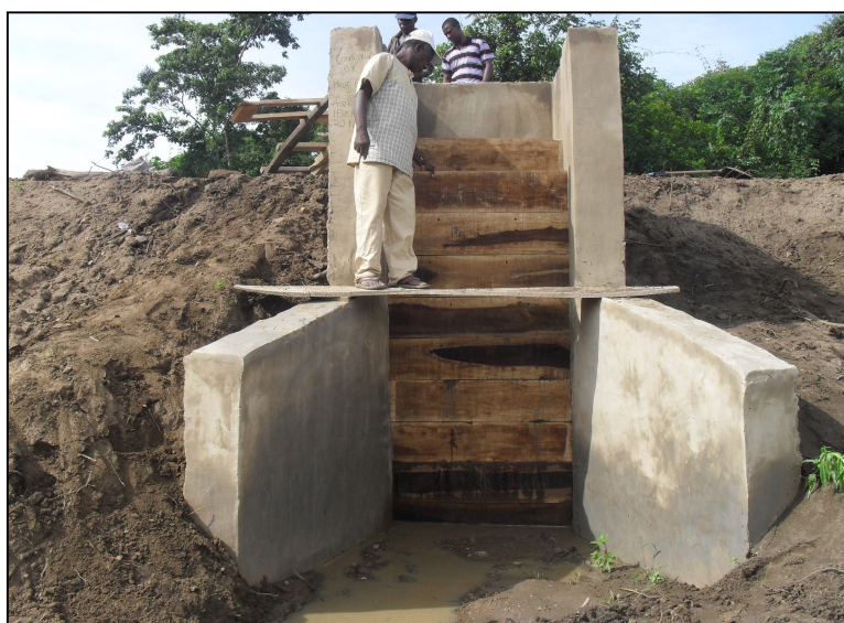
Plate 12: Construction of Monk at Opeji Courtesy. Prof. G.N.O. Ezeri et.al. (2010)
