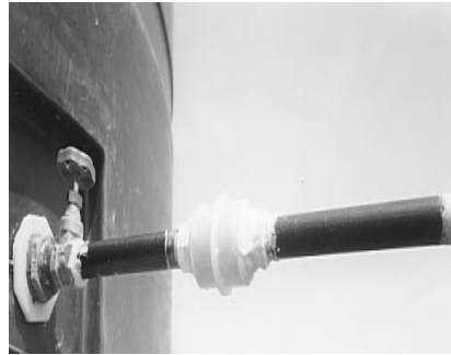
Figure 4: The low-cost secondary filter
