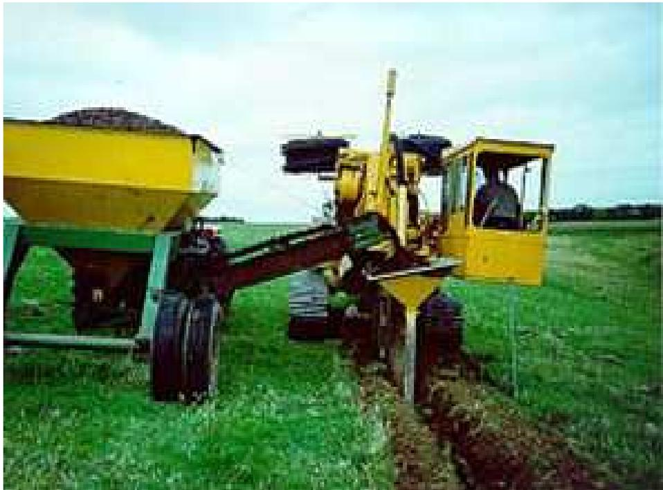
*Drainage trencher installing subsurface pipe drains*
