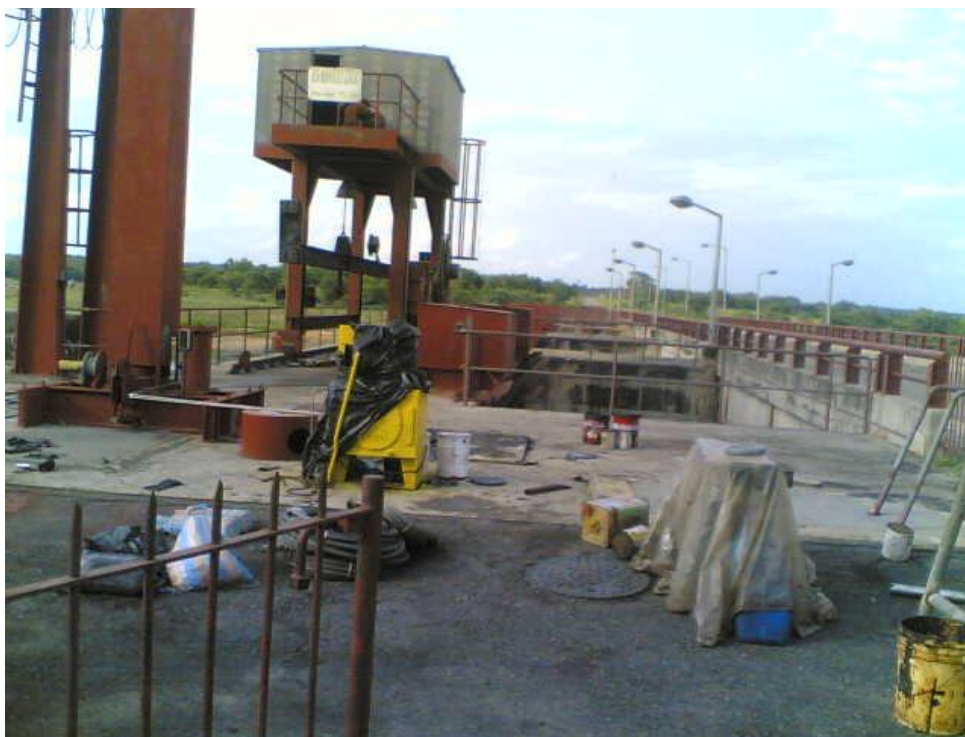
Fig. 3: On-going maintenance activity (May, 2010)
