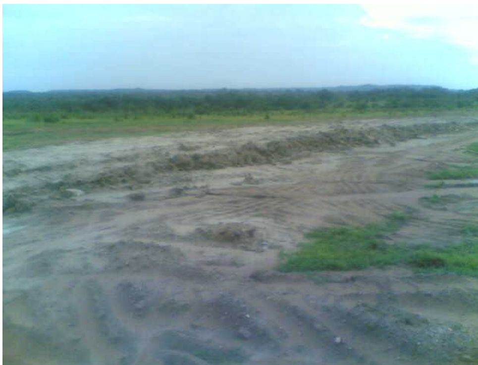
Fig. 4: Construction activity for expansion of irrigation scheme
