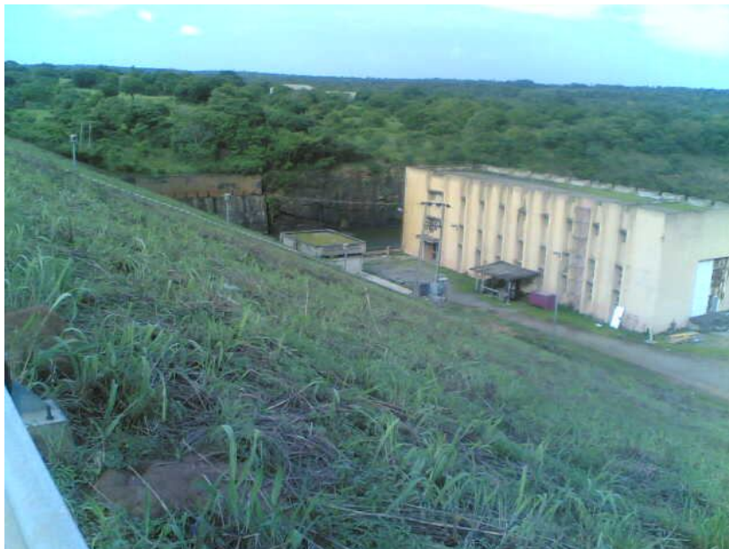
Fig 2: Oyan Dam Downstream Face showing Hydropower Building
