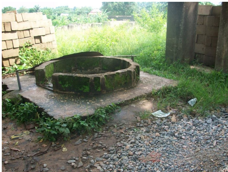
Fig. 2: Typical monitored well at Ugep
