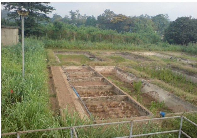
Plate 1: Reed bed prototype cells showing the irrigation pipe and the sludge drying beds
