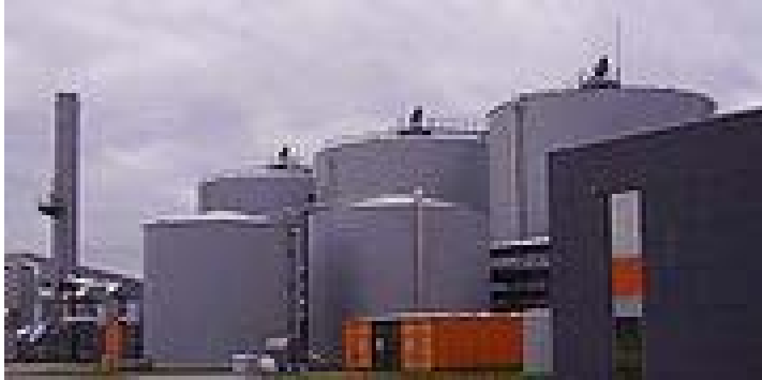
Anaerobic digestion component of Lübeck mechanical biological treatment plant in Germany, 2007
