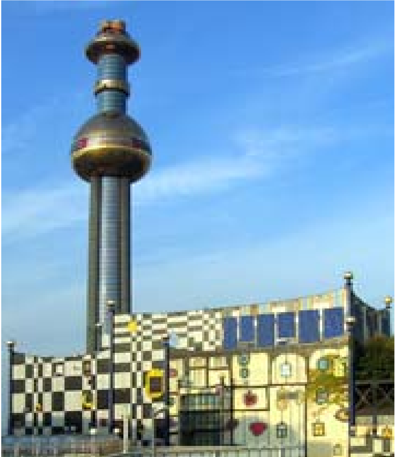
Spittelau incineration plant in Vienna.
