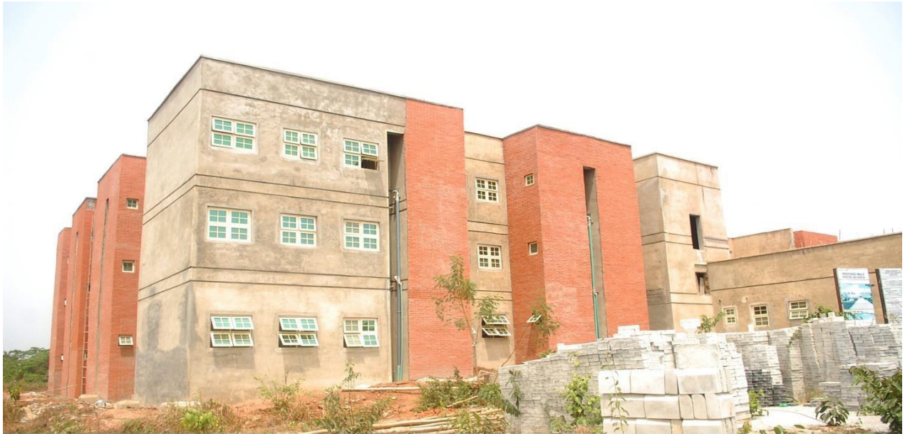
CONSTRUCTION OF MALE HOSTEL (BLOCK A) - FRONT VIEW
