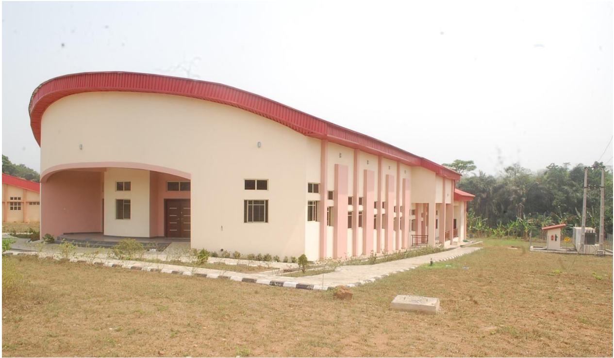
CONSTRUCTION OF 250 SEATER COMPUTER LABORATORY - FRONTAGE
