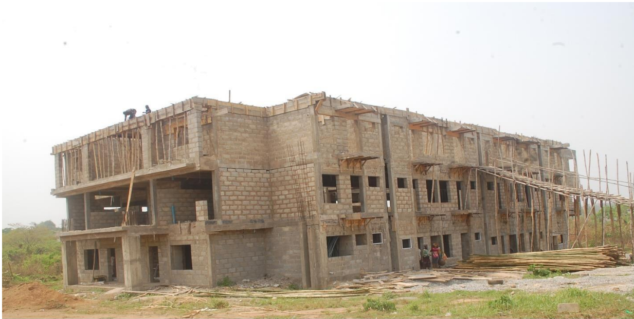
CONSTRUCTION OF POST GRADUATE STUDENTS HOSTEL (BLOCK A) - FRONTAGE
