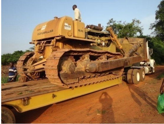
Arrival of the bulldozer
