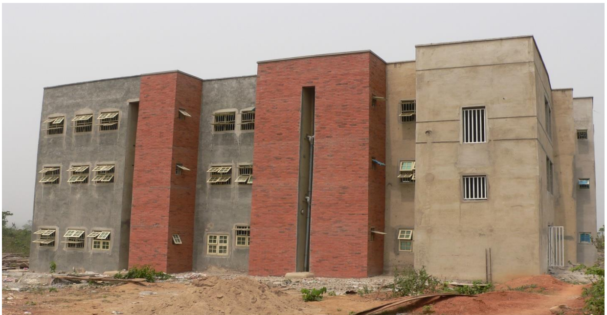
CONSTRUCTION OF FEMALE HOSTEL (BLOCK A) -FRONTAGE
