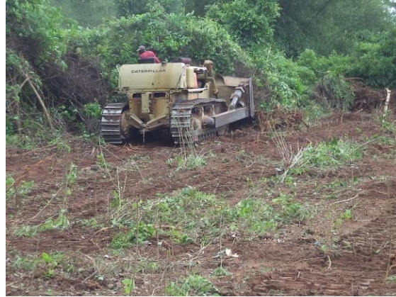
Bulldozer in action clearing
