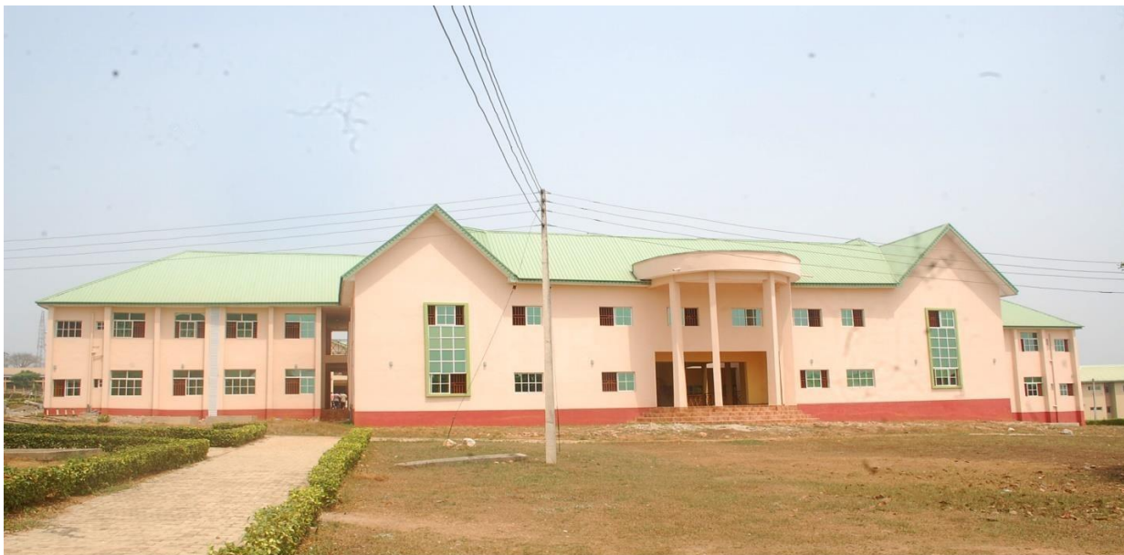
CONSTRUCTION OF COLLEGE OF FOOD SCIENCE AND HUMAN ECOLOGY (COLFHEC) PHASE II - FRONTAGE
