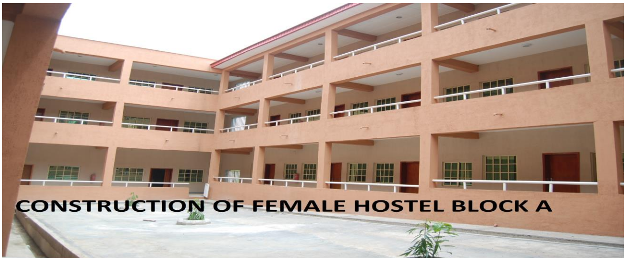
CONSTRUCTION OF FEMALE HOSTEL BLOCK A
