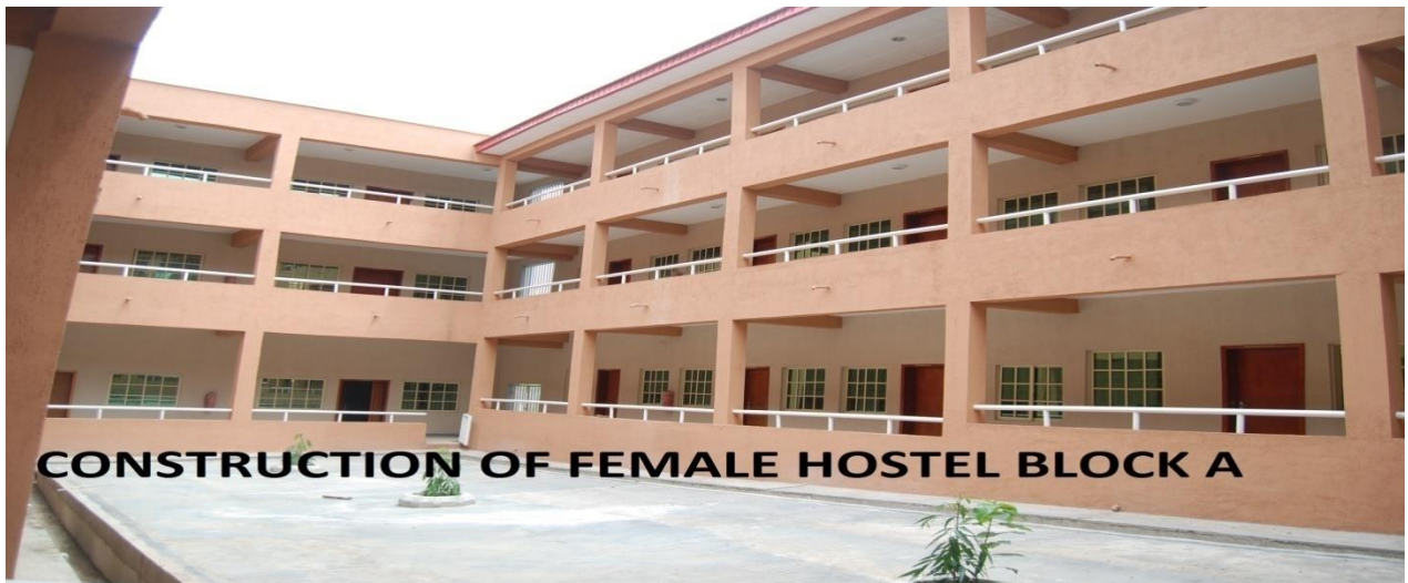
CONSTRUCTION OF FEMALE HOSTEL BLOCK A
