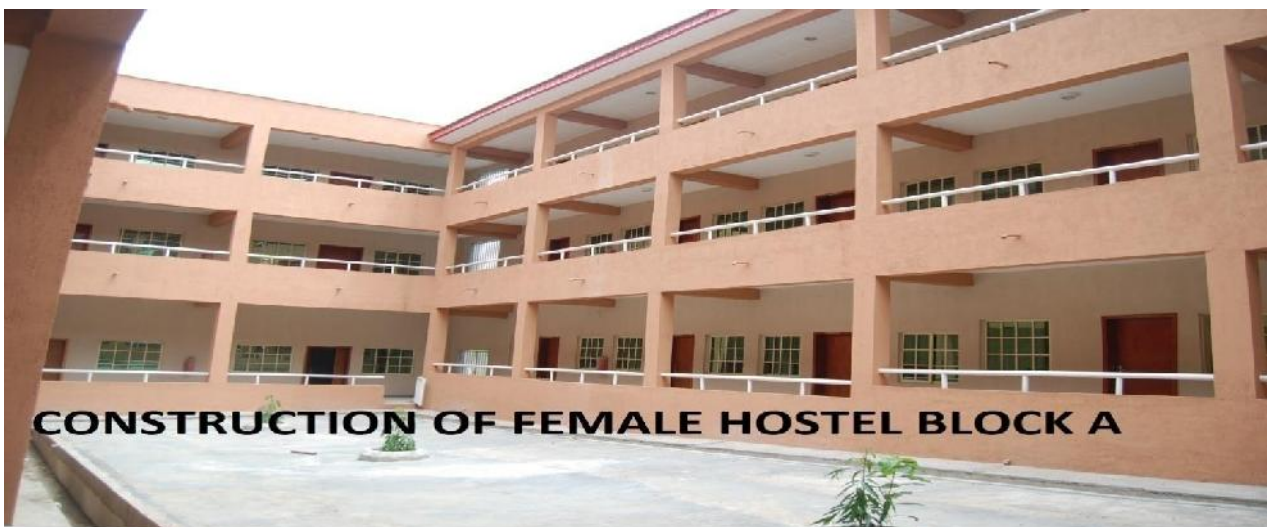
CONSTRUCTION OF FEMALE HOSTEL BLOCK A
