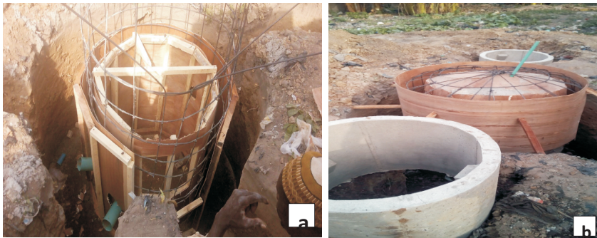
Plate 1. Construction of digestion dome.
