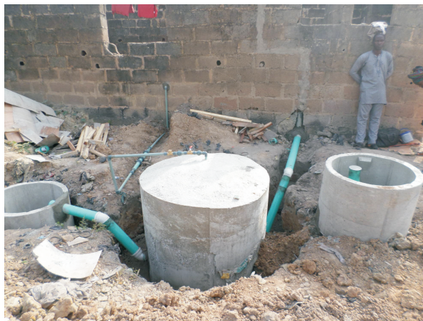
Plate 2: Biogas digester construction with pipe fixings
