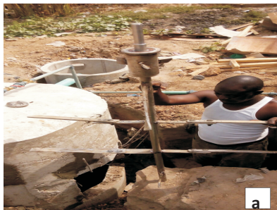
Plate 5: Stirrer constructed with antirust steel metal: a)- stirrer before installation and b)-stirrer after installation
