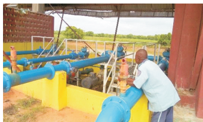
Fig. 41: Pump station for surface irrigation station.
