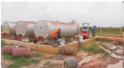
Figure 34: Fuel depot at field workshop to ease fuel supply to machines right on the field.
